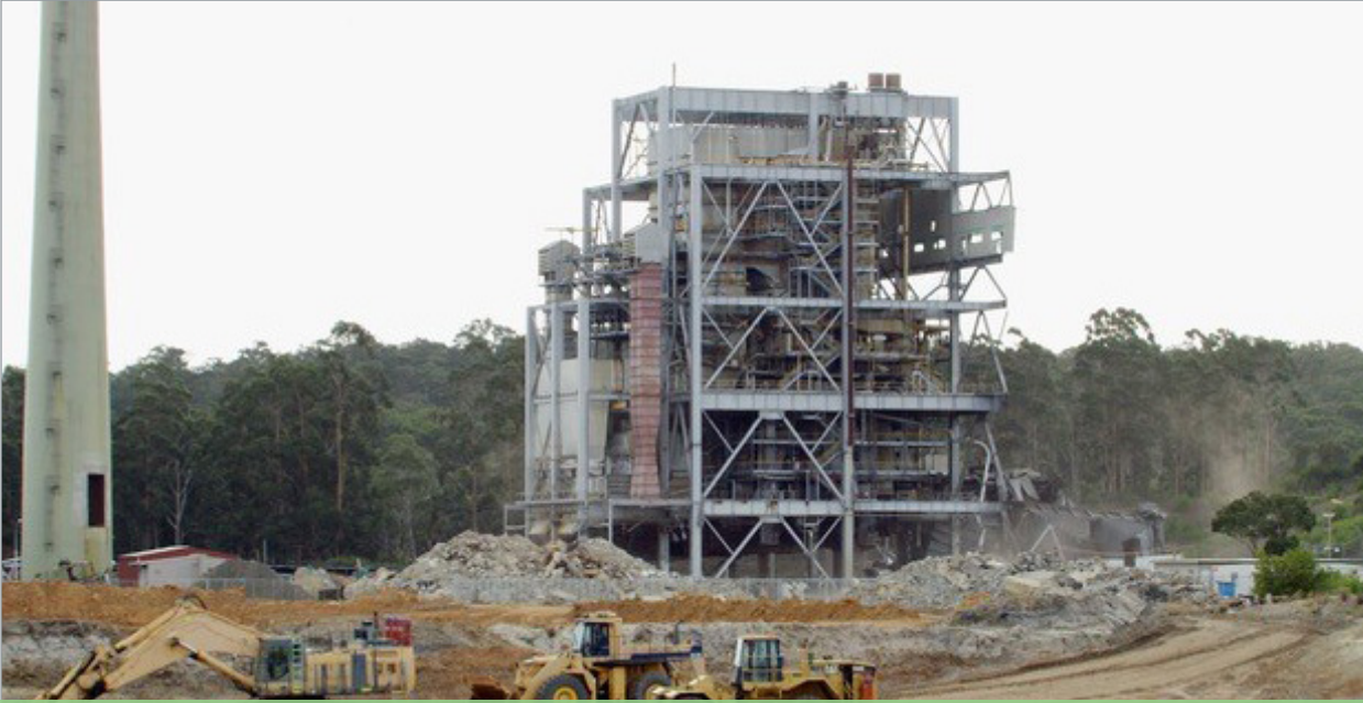
The remaining Anglesea Power Station structure
