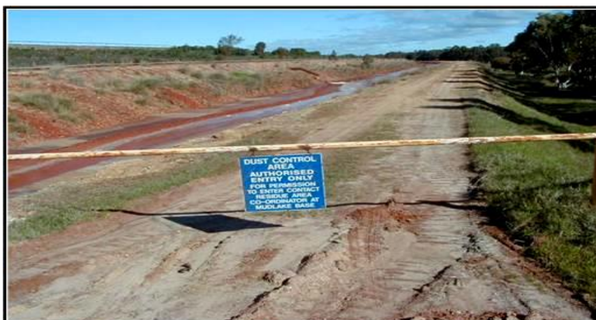
Figure 5: Less Trafficked Roads are Blocked off to Reduce Dust Emissions
