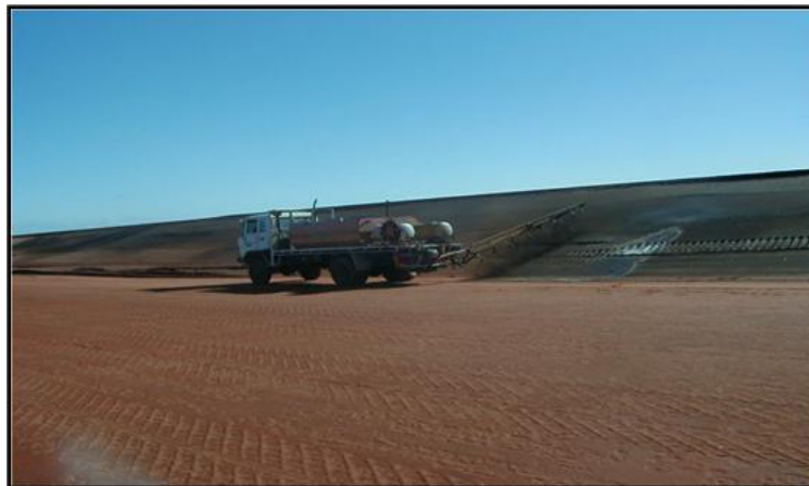
Figure 3: Bitumen Emulsion Being Sprayed to Reduce Dust Emissions from Embankment Walls
