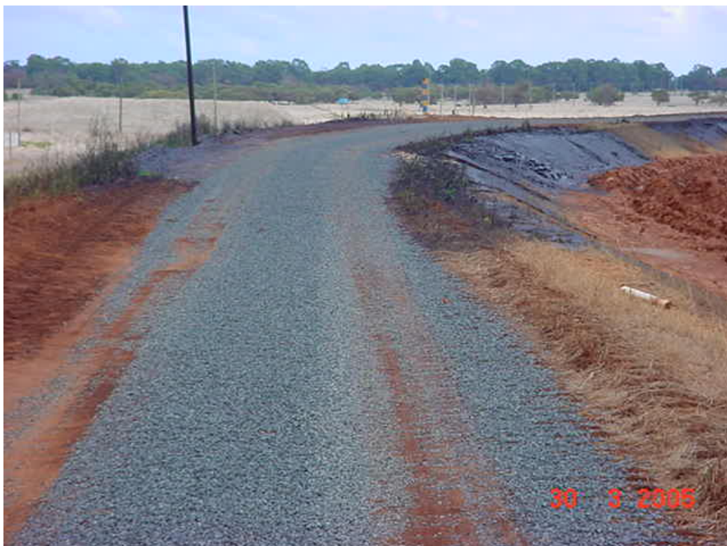
Figure 1.9 Blue metal covering on a road and bitumen coverage on embankment to minimise wind erosion
