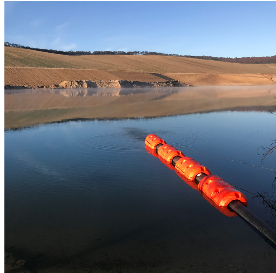
The groundwater enters the waterbody on the north-east wall via an above-ground pipeline from the groundwater bore.
