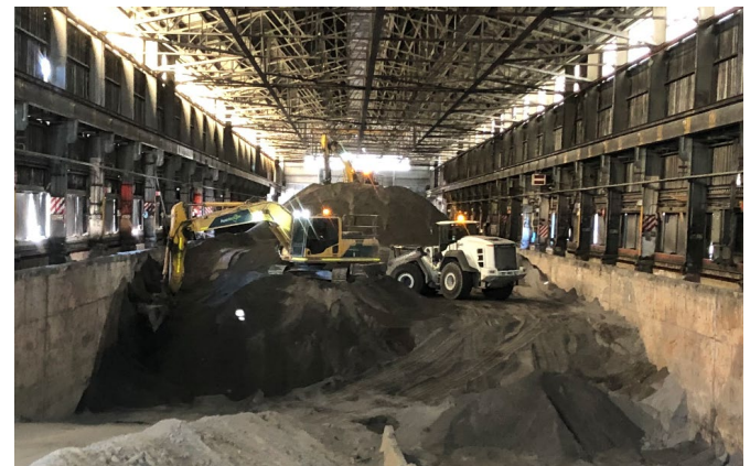
Above: Treatment of onsite materials
